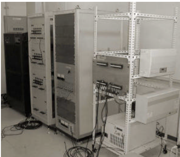
Fig.3 Installation situation of experiment equipment
