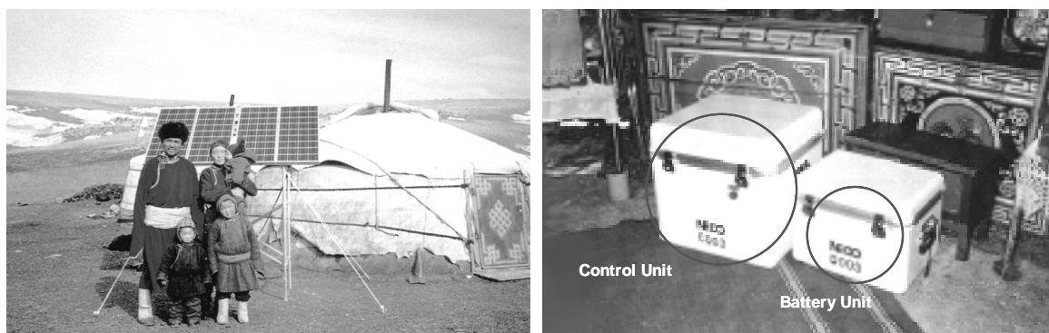
Fig.3 Typical SHS for Mongolian nomadic family with 200W PV modules
